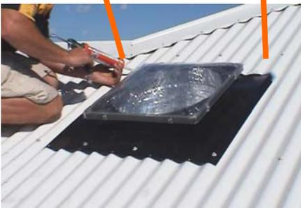
Using a Roof & Gutter Silicone, seal both corners on the high side of the Soaker Tray.
