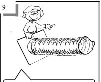
ALLOW SUFFICIENT LENGTH OF FLEXI-TUBE TO REACH FROM ROOF TO CEILING (REMEMBER TO ALLOW FOR BENDS IN FLEXI-TUBE). TAPE THE BOTTOM STAINLESS STEEL RING TO THE FLEXI-TUBE.
